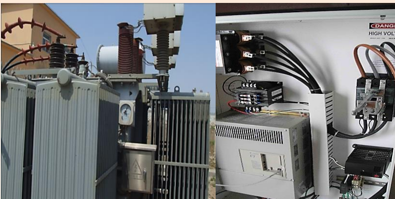
Utilisation of power compensation device and frequency conversion technology at the Yuedong oilfield
