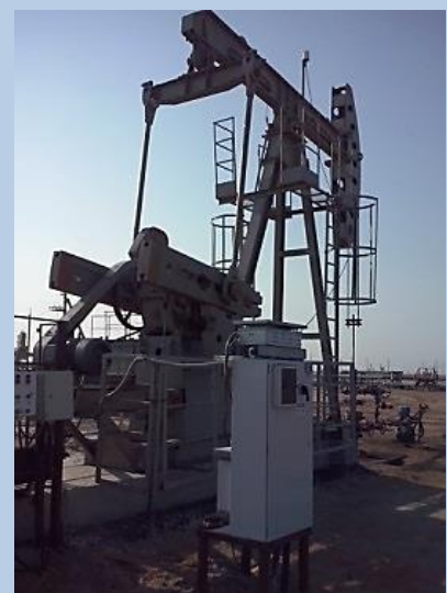
Variable-frequency controller with regular pump jacks at the Karazhanbas oilfield
